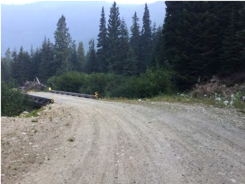
Approach from Right Bank when facing downstream
