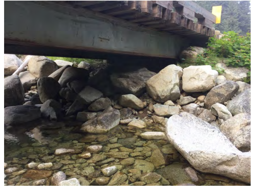
Left Bank Abutment when facing downstream
