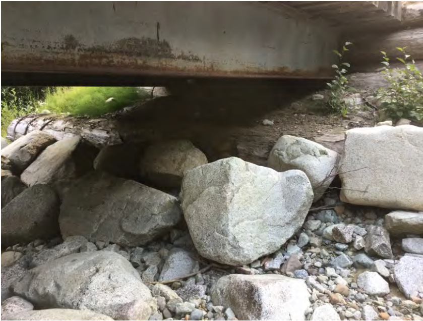
Right Bank Abutment when facing downstream
